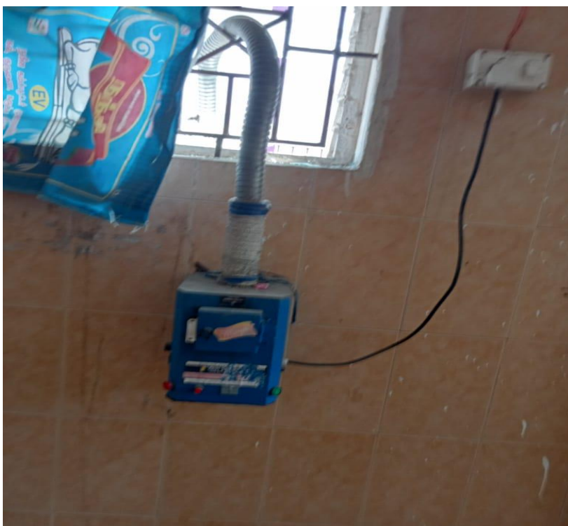
Sanitary Napkin Incinerator inside The Campus
